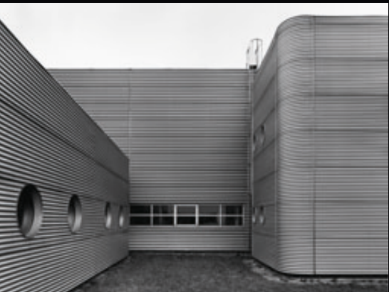
Factory Building, Nicholas Grimshaw, 1981/86
